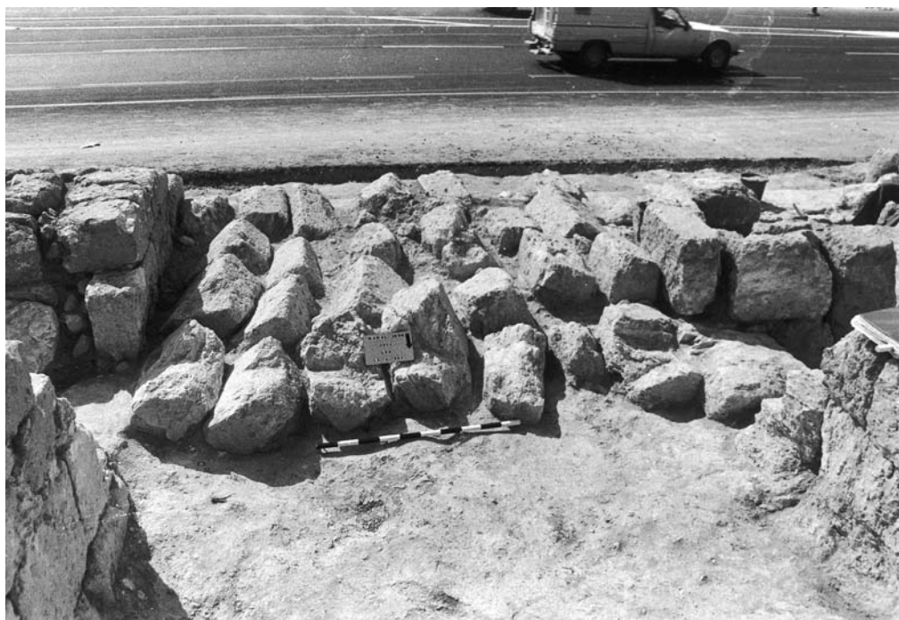
Fig. 3. Four rows of collapsed voussoirs from the barrel vaulting of the ceiling in Room XV, looking south.
